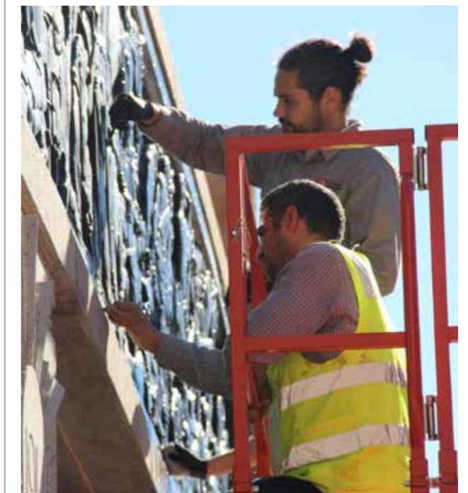
One of the bas reliefs undergoing conservation cleaning.
